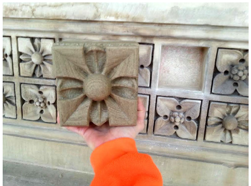
CLOCKWISE FROM TOP: WALL RESTORATION, BEFORE AND AFTER; CONSERVATION REPAIRS TO GROTESQUE; CLEANING AND CONSERVATION OF SCULPTURAL ELEMENT, BEFORE AND AFTER; DUTCHMAN REPAIR, DECORATIVE PANEL; CONSERVATION REPAIRS AND CLEANING OF GROTESQUE ELEMENT. ALL PHOTOS TAKEN ON THE WEST BLOCK, PARLIAMENT HILL, OTTAWA.
